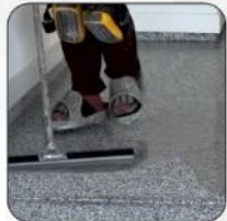
Grinding and Repair
